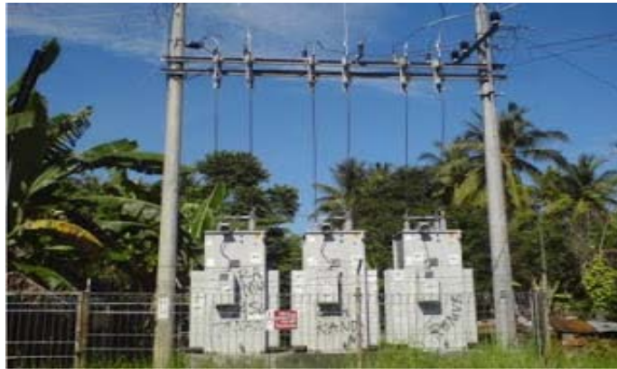
Gambar6.11 Auto Voltage Regulator
