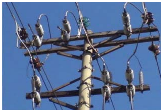
Gambar 6.13 Disconnecting Switch (DS)
