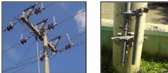
Gambar 6.14 Air Break Switch, Handle ABS w
